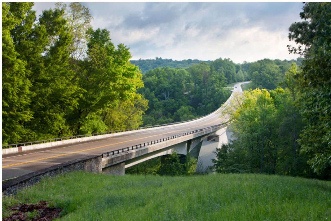
Vectors are used with surveying data for volume cut-and-fill dirt calculations for highway construction
