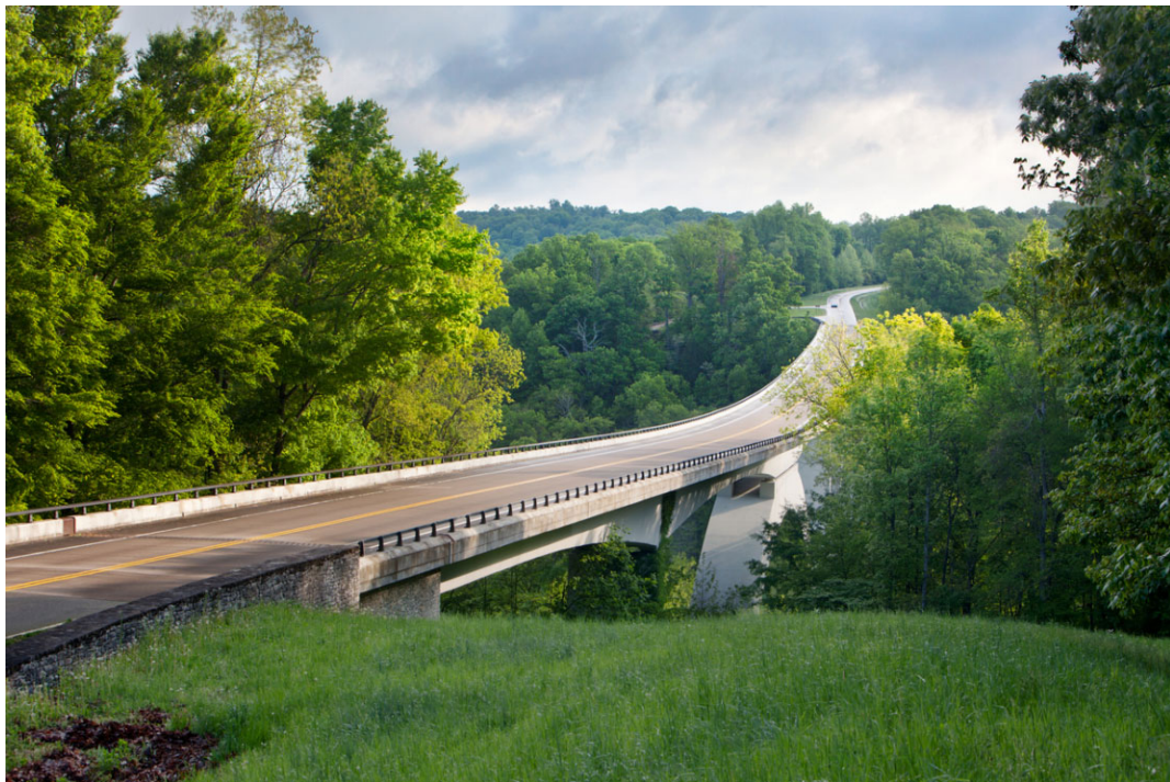
Vectors are used with surveying data for volume cut-and-fill dirt calculations for highway construction
